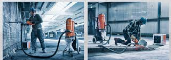
Dry cutting/drilling with an integrated dust collection device captures dust directly at the source. A dust extractor with the appropriate airflow and capacity for the application, also equipped with HEPA filters, takes care of the dust. The surrounding air is filtered through a portable air cleaner/scrubber 6–10 times/hour.
