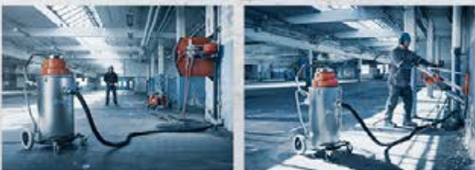
Wet cutting/drilling binds the dust with water directly at the source. The slurry collector connected to a slurry vac keeps the workplace clean.
