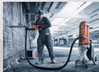
Dry cutting/drilling with an integrated dust collection device captures dust directly at the source. A dust extractor with the appropriate airflow and capacity for the application, also equipped with HEPA filters, takes care of the dust. The surrounding air is filtered through a portable air cleaner/scrubber 6–10 times/hour.
