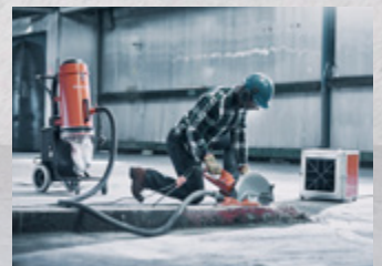
Dry cutting/drilling with an integrated dust collection device captures dust directly at the source. A dust extractor with the appropriate airflow and capacity for the application, also equipped with HEPA filters, takes care of the dust. The surrounding air is filtered through a portable air cleaner/scrubber 6–10 times/hour.
