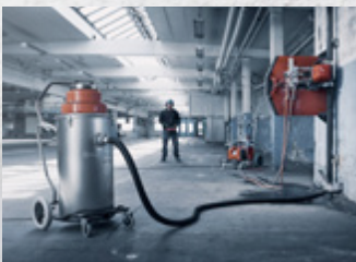
Wet cutting/drilling binds the dust with water directly at the source. The slurry collector connected to a slurry vac keeps the workplace clean.
