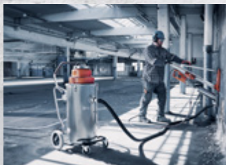
Wet cutting/drilling binds the dust with water directly at the source. The slurry collector connected to a slurry vac keeps the workplace clean.
